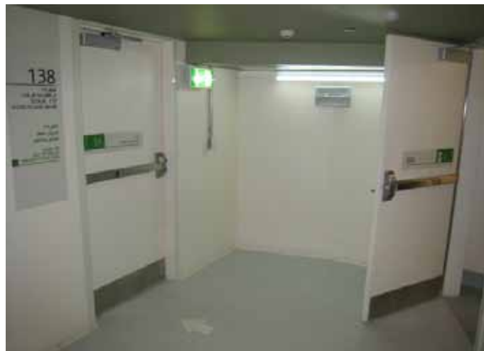
Figure 4. Entrance into the 2 hour protected refuge floor area at floor 138 in the Burj Khalifa (Source: Dan O'Connor)
