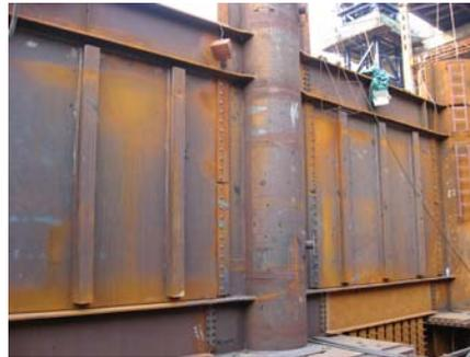
**Fig. 4.** Buckling Restrainted SPSWs
