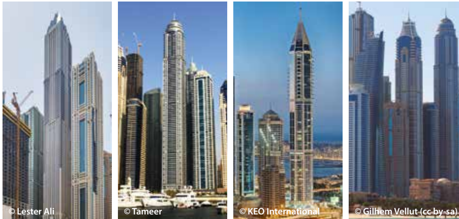
Figure 4. Examples of supertall residential buildings in Dubai Marina in Group A: (from the left) Marina 101 (425 m), Princess Tower (414 m), 23 Marina (392 m), and Elite Residence (381 m).
