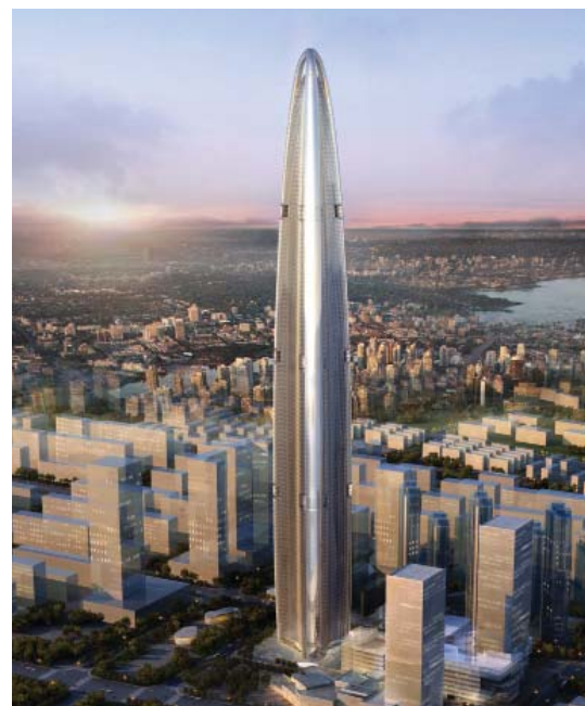
图5. 武汉绿地中心独特的楼板槽有助于减少涡流 © AS + GG Architects
