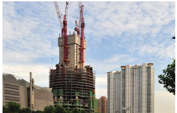
Figure 5. Integral steel platform 图5. 整体钢平台
