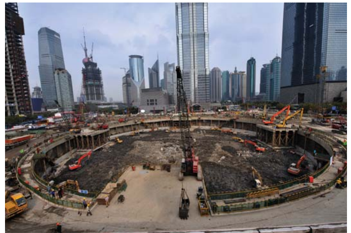
Figure 2. Excavation of the foundation pit of the tower 图2. 主楼基坑开挖
