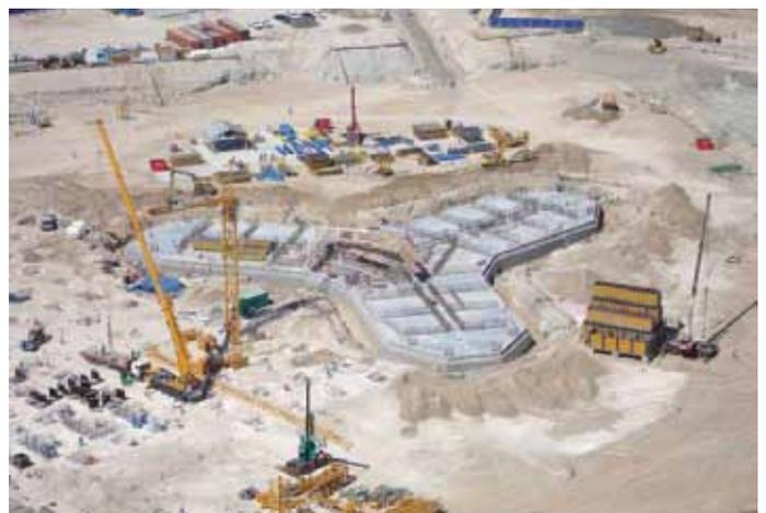
Figure 6. The concrete base for the tower.
