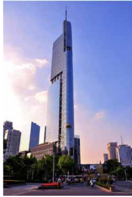
Figure 2. Nanjing Greenland Square Zifeng Tower 图2. 绿地南京紫峰大厦
