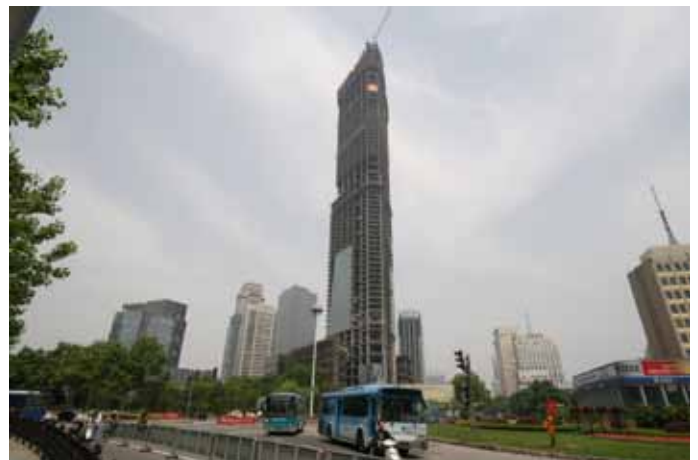
Figure 6. Nanjing Zifeng Tower under construction 图6. 施工中的南京紫峰大厦
