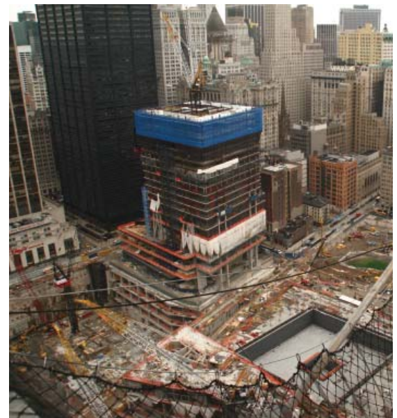
Figure 6. Tower 4 under construction © Jan Klerks
