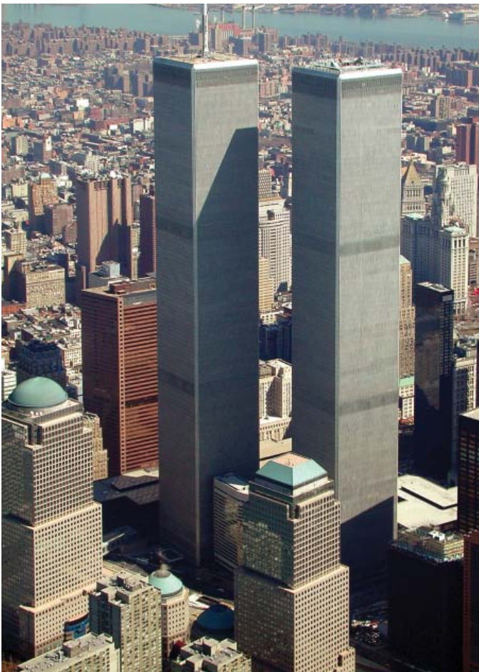
Figure 5 The Twin Towers © Scott Murphy
