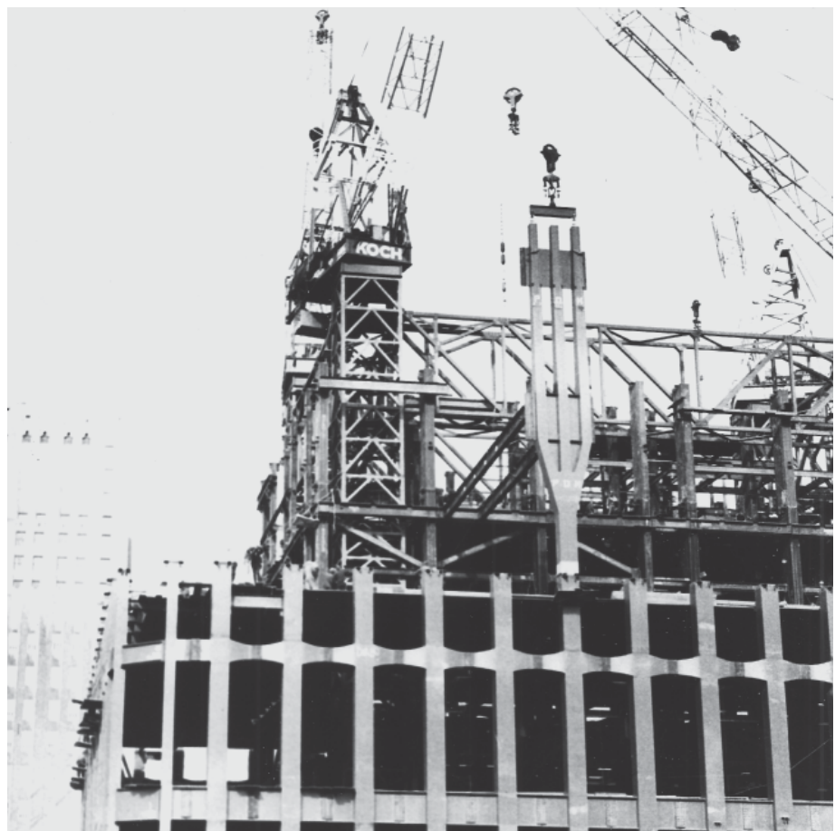
Figure 1. Former World Trade Center load bearing wall © CTBUH Ramsey Collection
