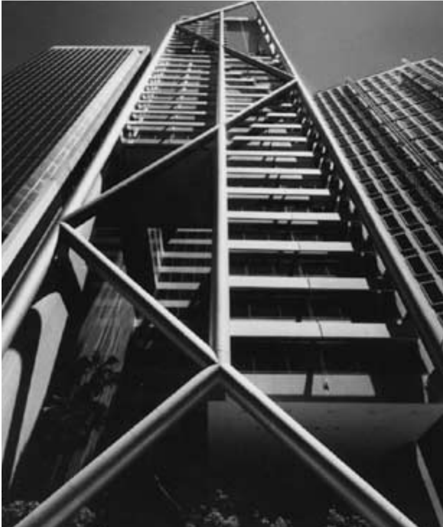
15.14a. Capita Centre, Sydney, 1989. Architect and photo: Harry Seidler.
