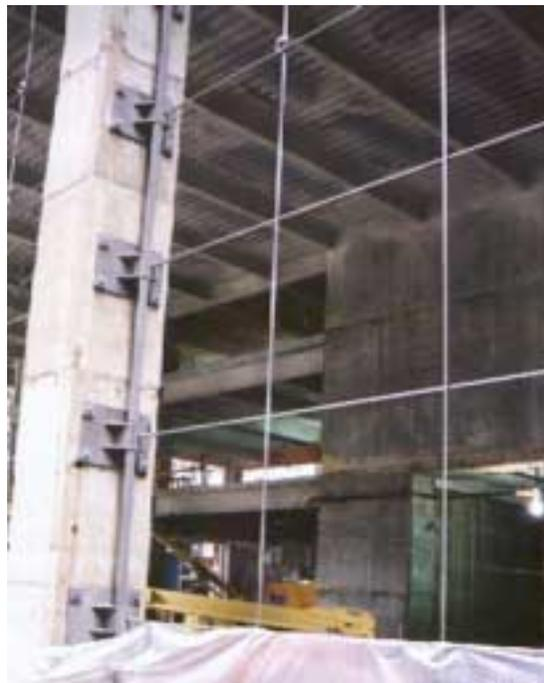
Fig. 3 Pretensioned cable grid in the south wall (courtesy of Joshua DeYoung)
