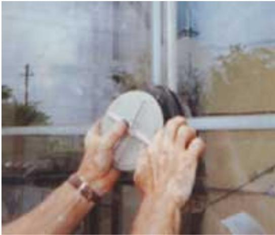
Fig. 4 Installation of a mock-up node in the net wall (courtesy of Lohan Associates)
