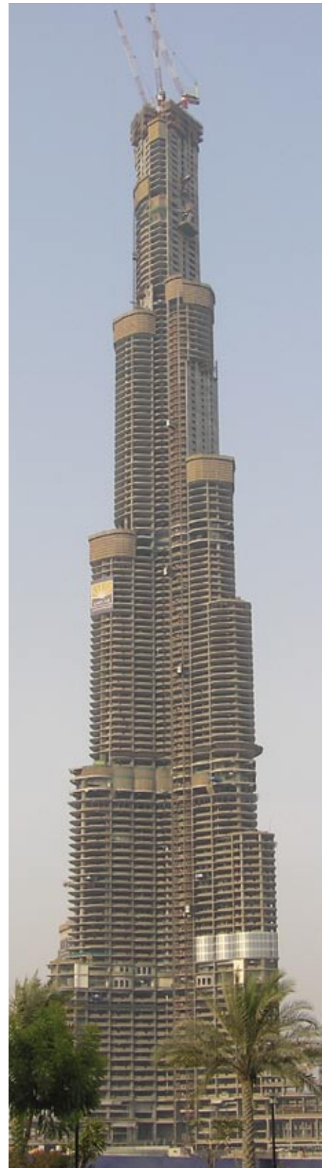
Fig 1. Burj Dubai under construction
