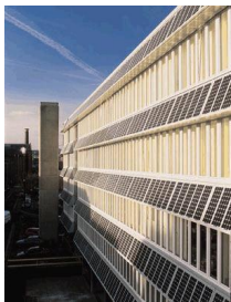
Figure 2, Northumberland building, PV rain screen block at the University of Newcastle. The installation provides 32,000kwh/y
