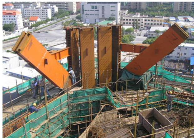
Figure 6. The diagonals of the mega-structure, formed from welded boxes of structural steel.
