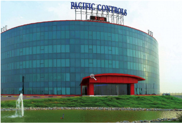
Figure 3. Pacific Control Headquarters – the first LEED platinum-rated building in the Middle East. [Source: www.pacificcontrols.net ]
