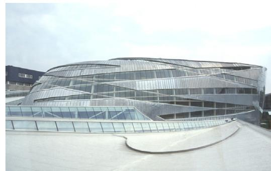
**Fig. 4.** Ribbon shaped glass zones cross the roof of the new town hall of Alphen aan de Rijn (NL)
