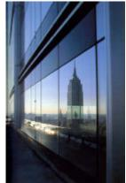
Fig. 2. Photovoltaic Spandrel Panel, Four Times Square
