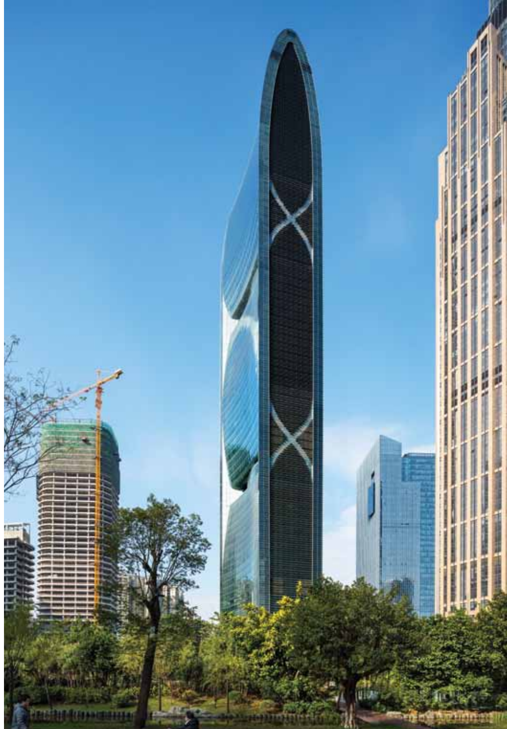
Figure 2. Pearl River Tower, Guangzhou.
