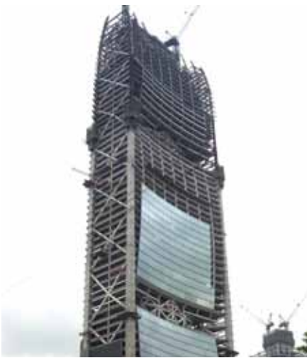
Figure 3. Lateral-load-resisting structural system.
