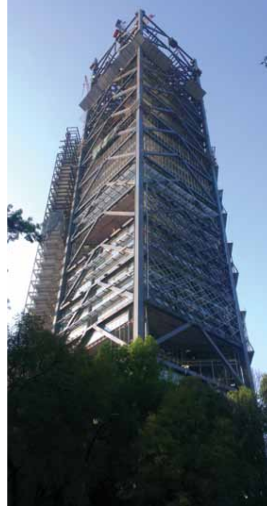
Figure 11. Construction photo of Torre BBVA Bancomer, January 2014.
