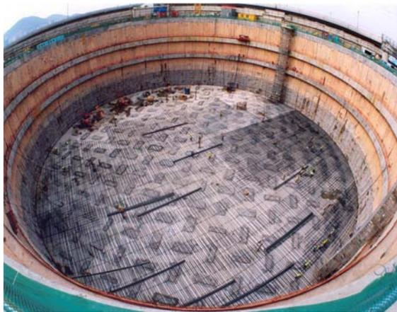
Fig. 8. Pile Layout within Cofferdam
