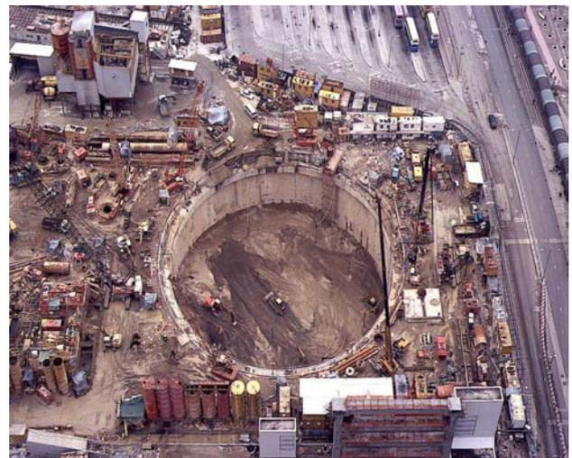
Fig.3. Excavation within the temporary cofferdam
