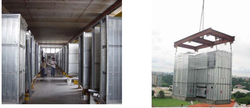
Figure 4: HDB's Prefabricated Boxed-Toilet
