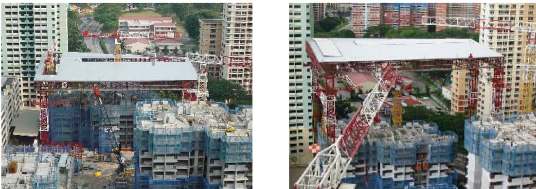
Figure 6: Automatic Building Construction System (ABCS)
