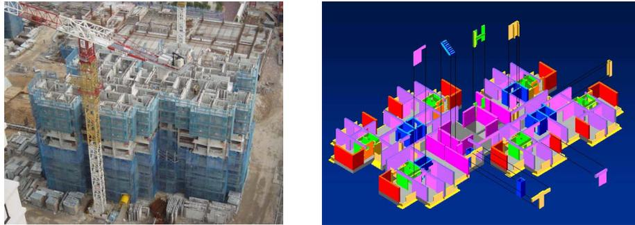
Figure 2: Fully Precast System used for super high-rise construction
