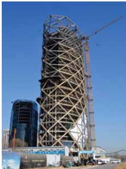
Figure 11. The Poly International Plaza, Beijing, employs a diagrid system using concrete-filled tubes that vary in diameter and thickness from  $\varnothing 1.3$  m, 50 mm thickness at the base to  $\varnothing 0.7$  m, 20 mm thickness at the top. Alternate floors are connected to the diagrid to create tensile connections between the nodes. Intermediate floors are hung from the floor above.
