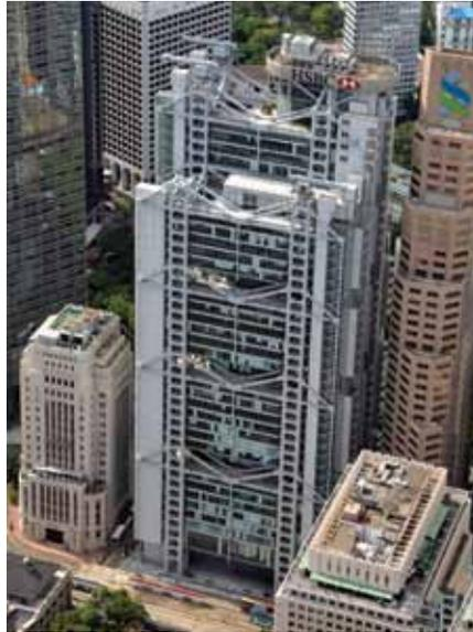
Figure 9. In 1985 the Hong Kong and Shanghai Bank by Foster + Partners launched the use of highly expressive structure and prefabricated components into the realm of tall building design.
