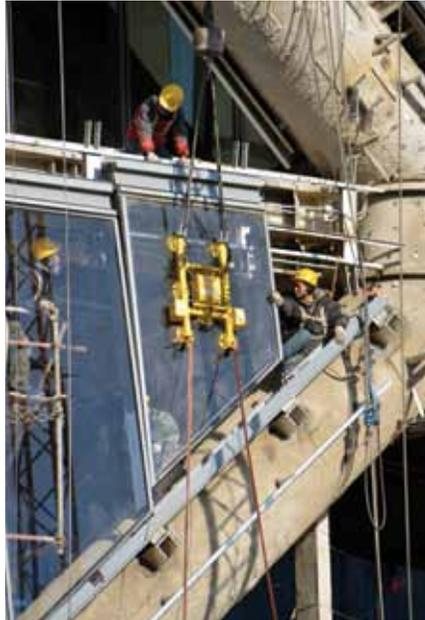
Figure 13. Workers install the glazing that will form the double façade system on the Poly International Plaza. The coordination of such complex geometries is possible only through the advancements of BIM systems.
