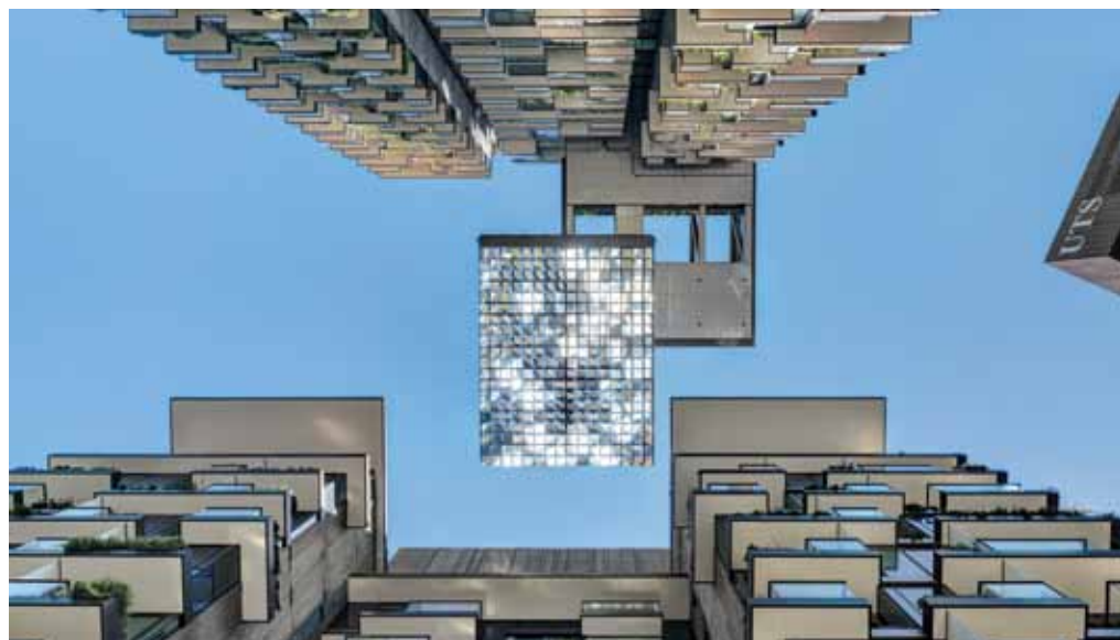
Figure 7. View looking up at the heliostat reflectors hanging from the cantilevered sky garden.
