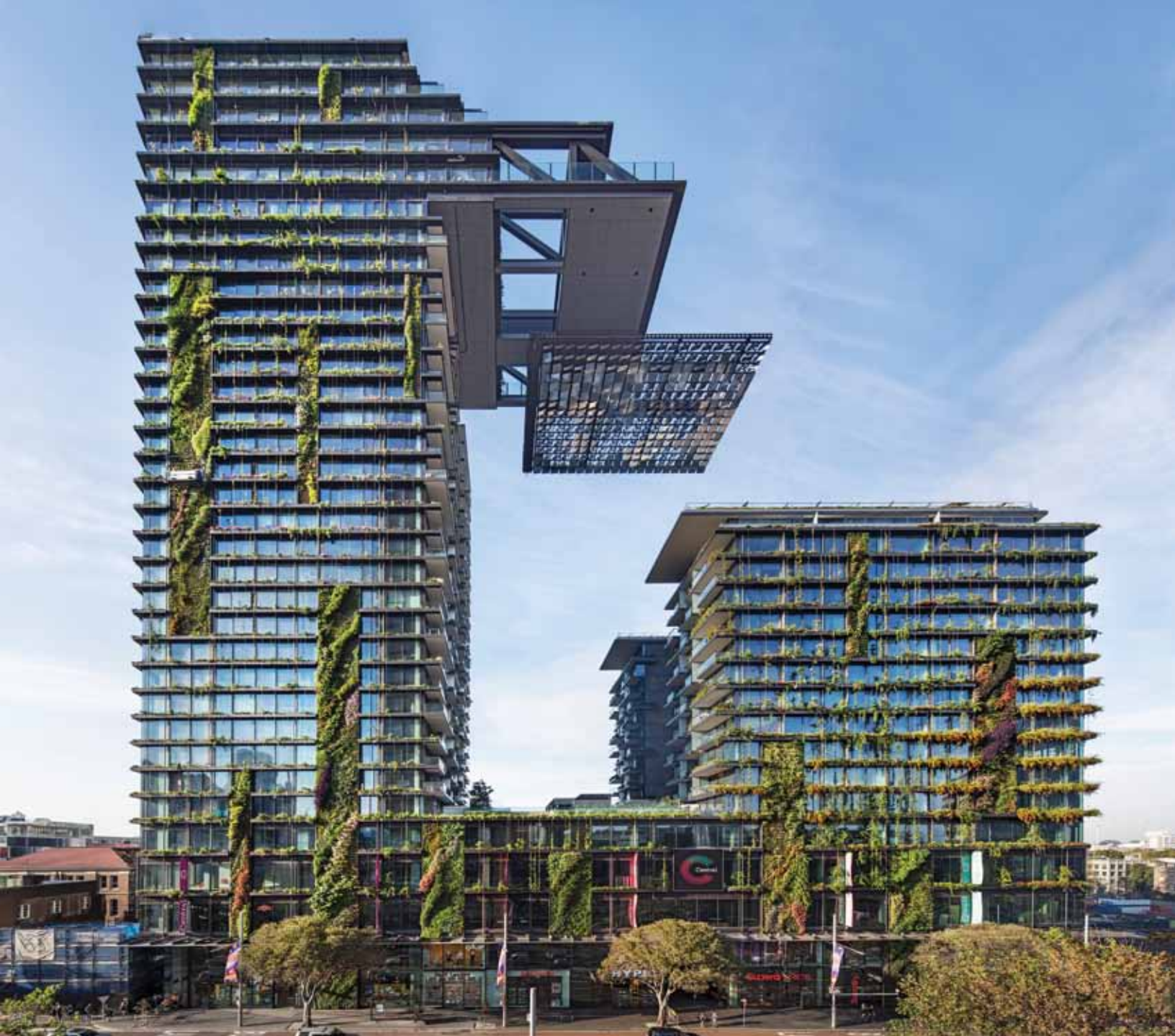
Figure 2. One Central Park, Sydney – overall view of tower from northwest.
