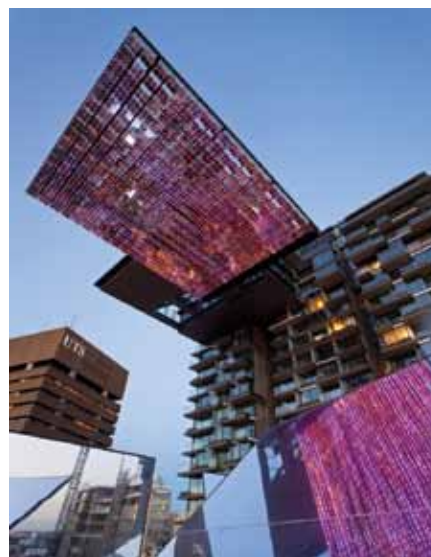
Figure 4. Heliostats on roof top and the cantilevered heliostat reflectors. © Simon Wood Photography
