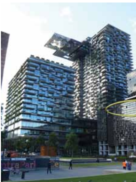
Figure 6. View from southwest. © Richard Braddish
