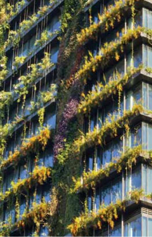
Figure 3. The vertical gardens maintained by the hydroponic system.
