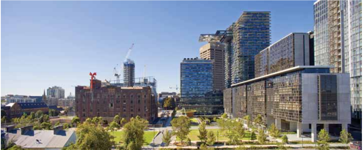
Figure 5. One Central Park public park. © Simon Wood Photography
