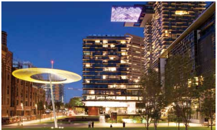
Figure 9. Heliostat reflectors at night.
