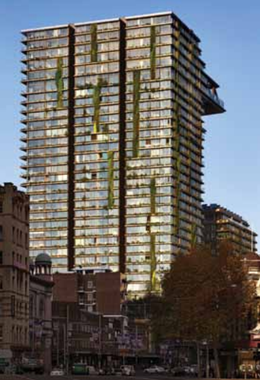
Figure 11. Deep vertical slots carved into the building to allow light and air.
