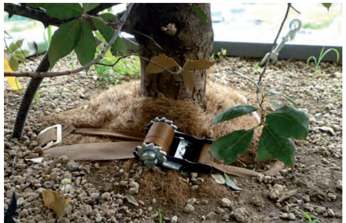
Figure 6. Anchoring System Of The Root Ball
