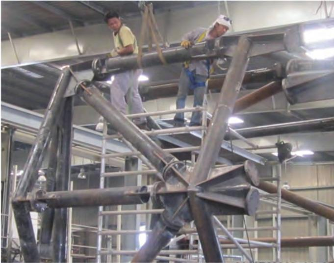
Figure 4. structure pre-assembly in the steel workshop (source AGC-A)
