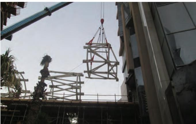
Figure 5. Erection of bridge module (source: AGC-A)
