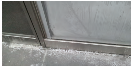
Figure 2. Condensation on backside of glass in a shadow box. (Source: Neil McClelland HOK) 图2. 阴影框背面玻璃上的凝结。(来源: 尼尔·麦克莱兰HOK公司)
