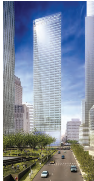
Figure 4. Seven World Trade Center. (Source: Skidmore, Owings & Merrill LLP) 图4. 世贸中心7号 (来源于Skidmore, Owings & Merrill LLP)
