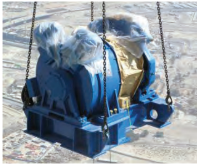
Figure 1. SkywayTM machine being lifted to the top of Burj Khalifa building in Dubai, (Source: Otis Elevator Company)
