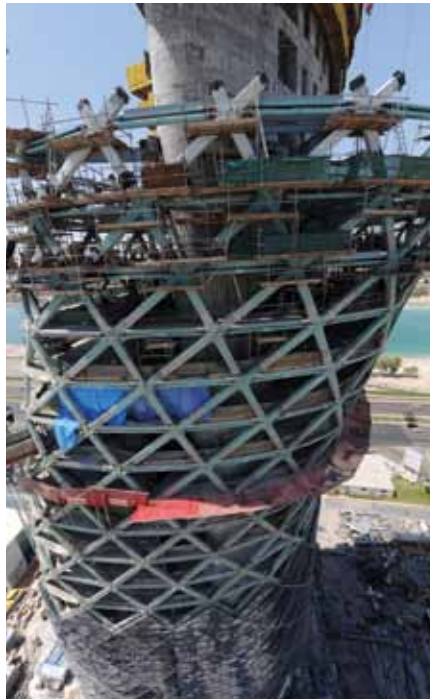
Figure 7. External diagrid structure © ADNEC
