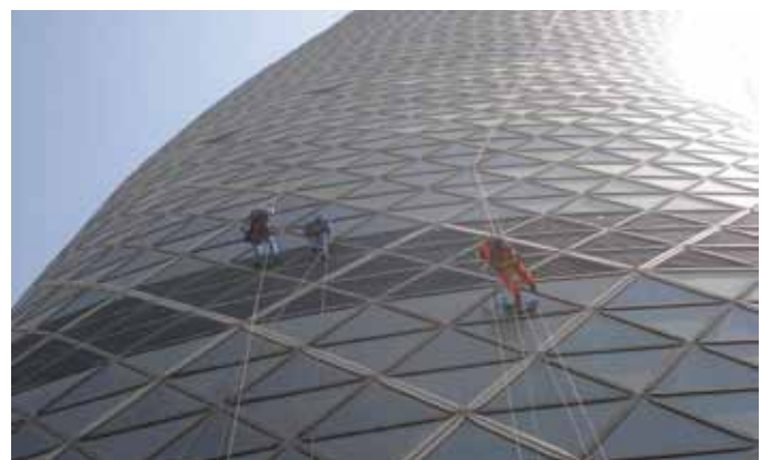
Figure 10. Façade maintenance via abseiling from the outside © ADNEC
