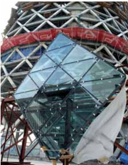
Figure 9. Curtain wall diamond-shaped panels © Jeff Schofield
