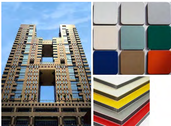
Figure 4.12. Aluminum composite panel for curtain wall cladding (Sky City, Taiwan, China) 图4.12. 铝塑板外墙 (台湾天空之城)
