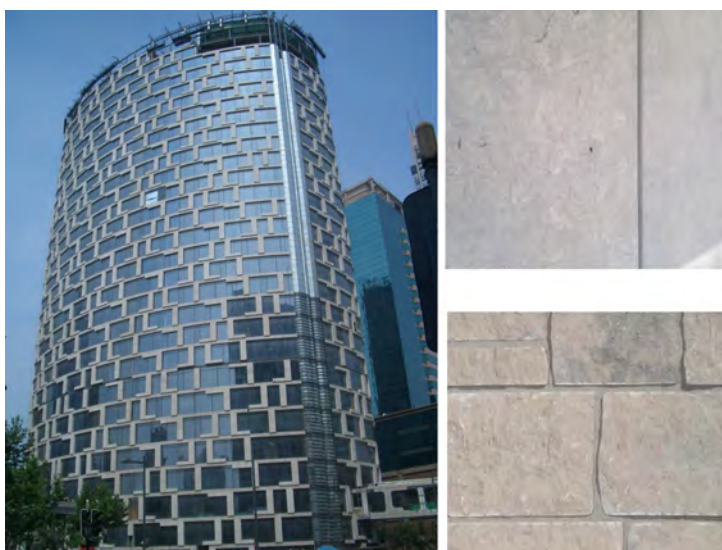
Figure 4.10. Building stone cladding (Building near Xintiandi, Shanghai) 图4.10. 石材外墙 (中国新天地项目)
