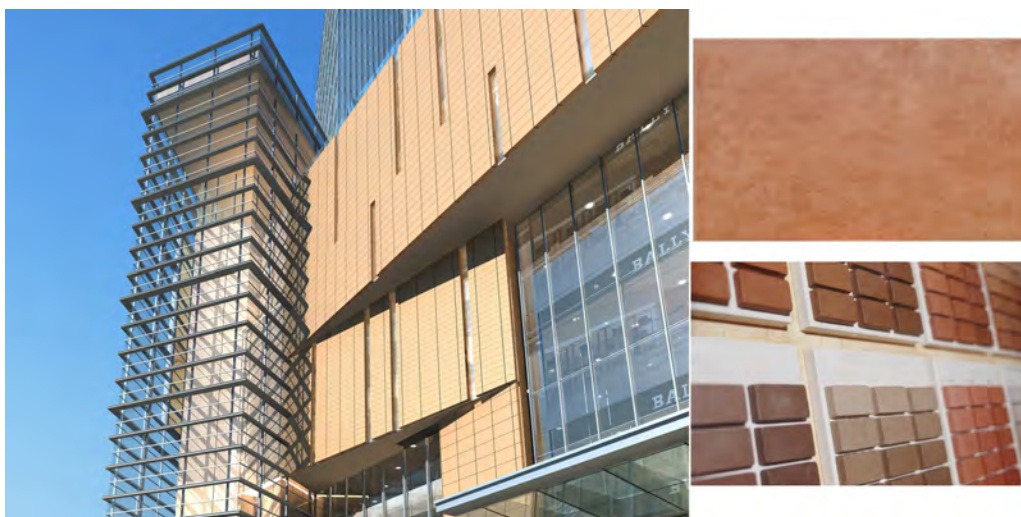
Figure 4.13. Curtain wall cladding with terra cotta (Beijing Huamao Center, China) 图4.13. 陶土板外墙 (中国北京国贸中心)
