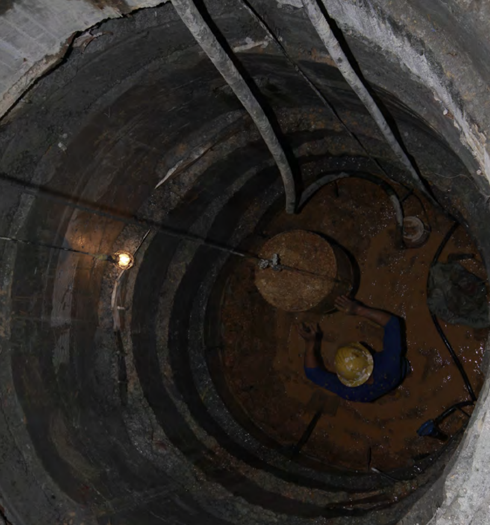
Figure 2.15. Construction process of the piles (Source: Ping An) 图 2.15 桩施工过程 (来源: 平安)
