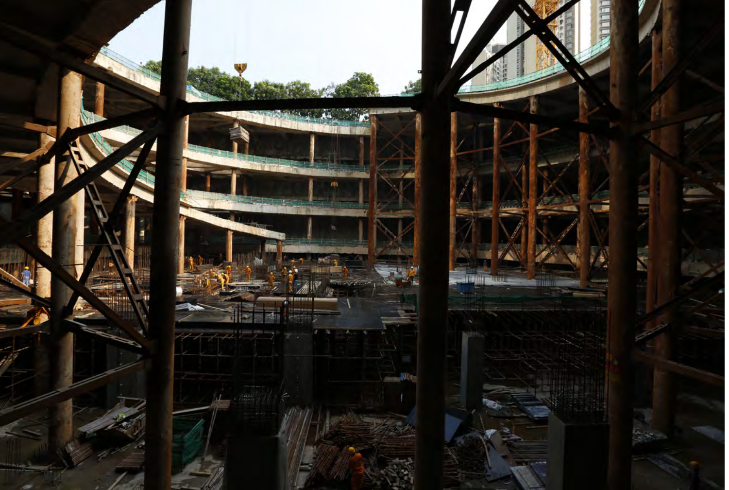
Figure 6.11. The structural support for the parking garage and weather proofing to prevent water leakage. (Source: Ping An) 图6.11. 停车场的结构支撑以及防渗水的耐候件 (来源: 平安)
