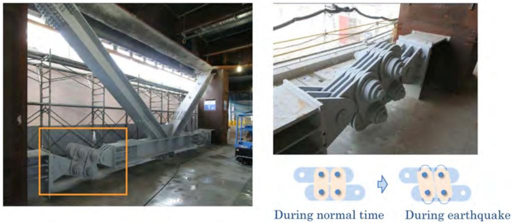
Figure 28. Appearance of rotational friction damper.
