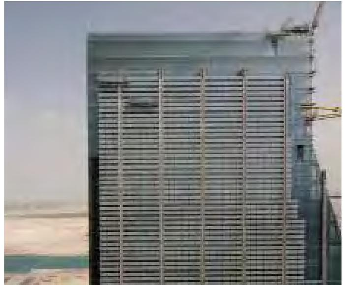
Figure 7. Construction photo of Sowwah Square with operable shades in closed position (Source: Goettsch Partners)
