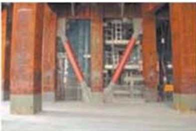
Figure 5. Toranomon Hills response-control devices.
