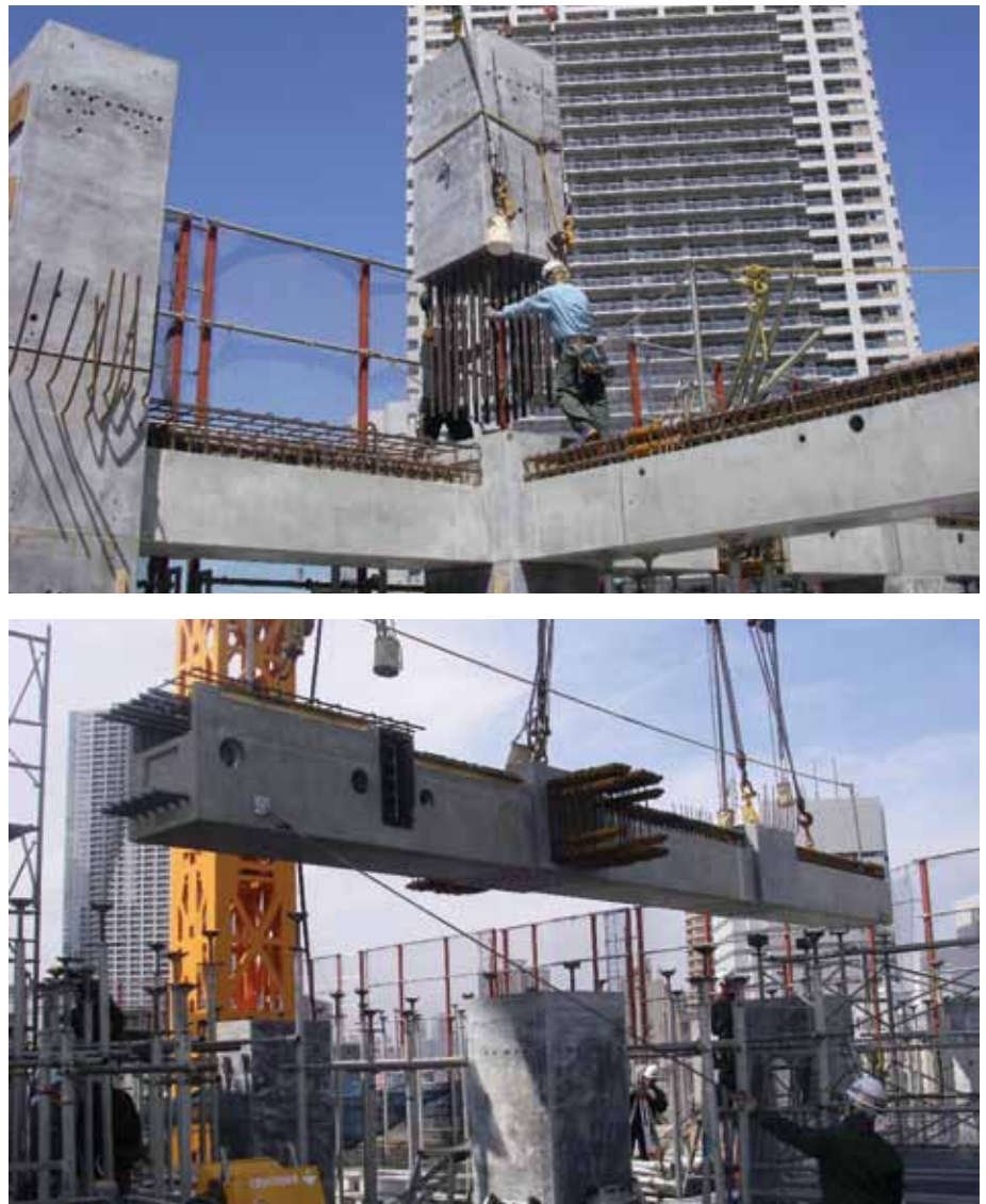
Figure 14. V column and LR beam used for LRV Method. © Obayashi Corporation
