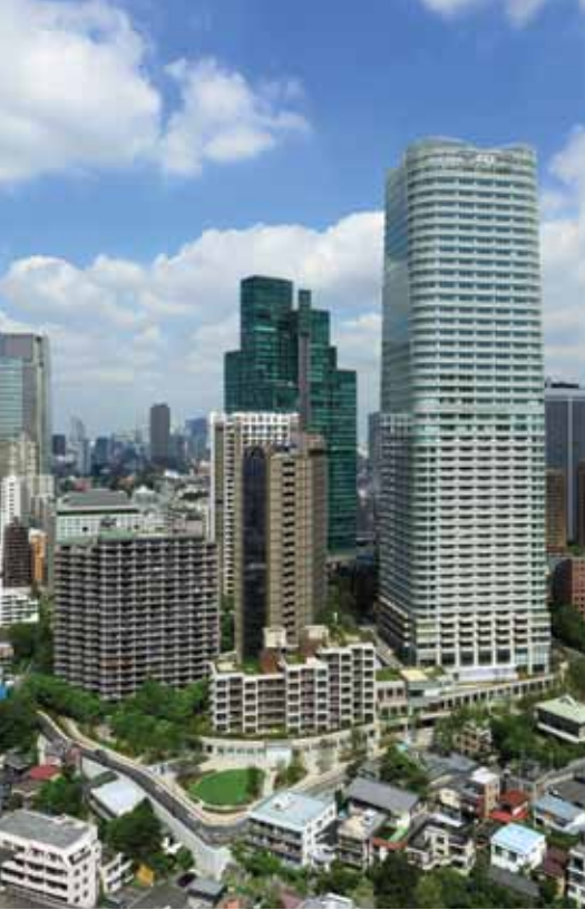
Figure 10. Ark Hills Sengokuyama Mori Tower, Tokyo. © Mori Building
