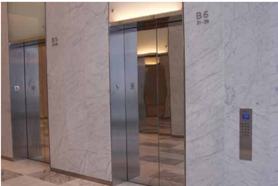
Top: 7 World Trade Center, New York. Source: UTC Building & Industrial Systems
