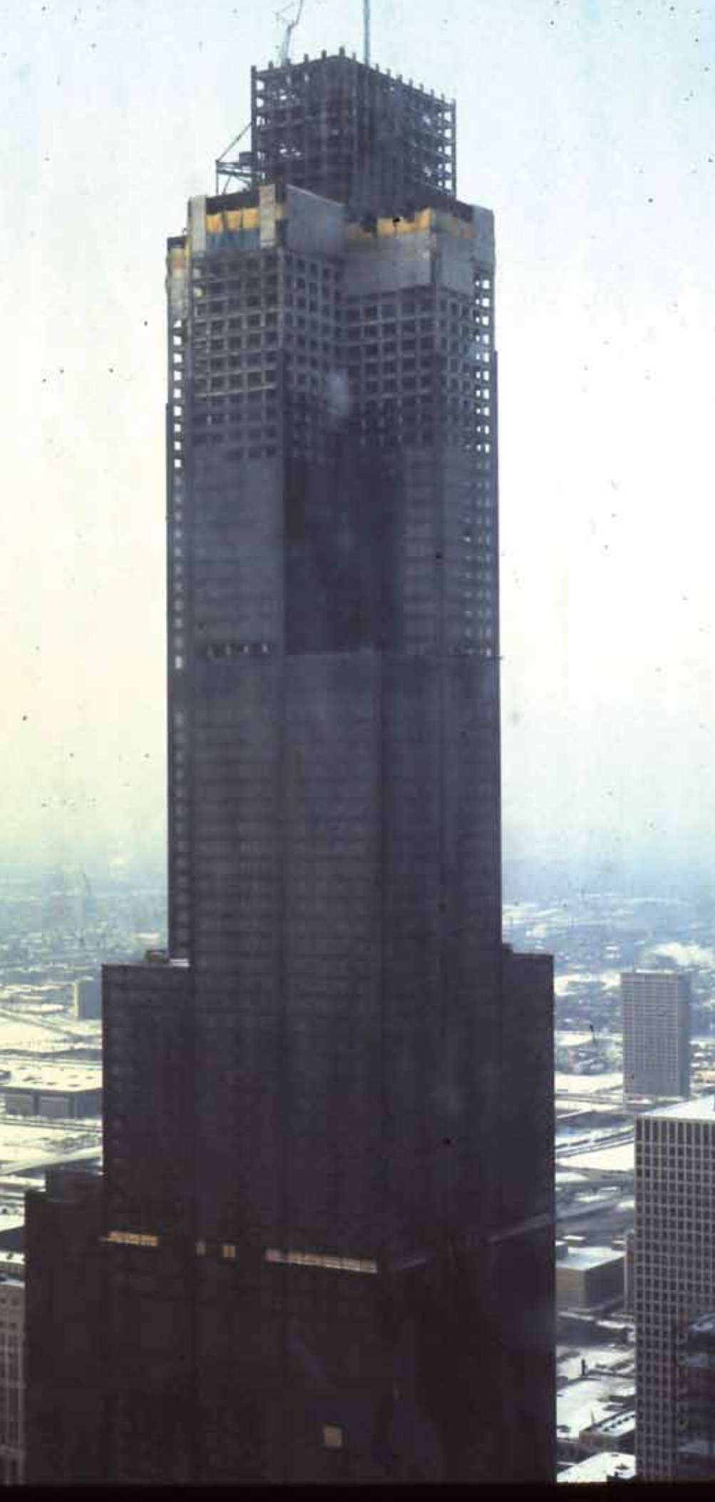
Left: Willis (then Sears) Tower, Chicago, under construction circa 1973. (cc-by-sa) Steveboerger
