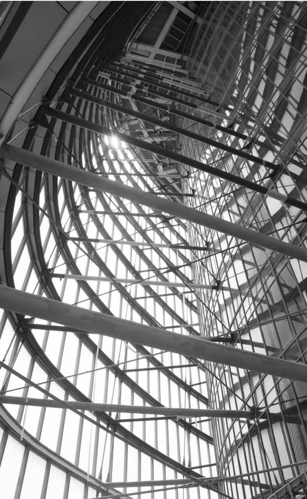
also represents significant achievements in structural safety and cost savings. It shows the elegance and fashionable characteristics of Shanghai by twisting the outer enclosure by 120 degrees while spiraling up. Through wind-tunnel tests, its designers determined that we know that the wind load could be reduced 24 percent, which is quite considerable in a city that suffers from typhoons every year, saving 20,000 metric tons of steel in the process.
