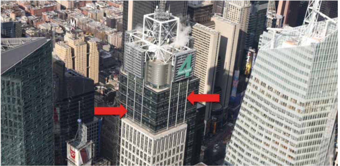
Figure 5. The photovoltaic cells at 4 Times Square. Arrows indicate approximate location of building-integrated photovoltaics. (Source: The Durst Organization)
