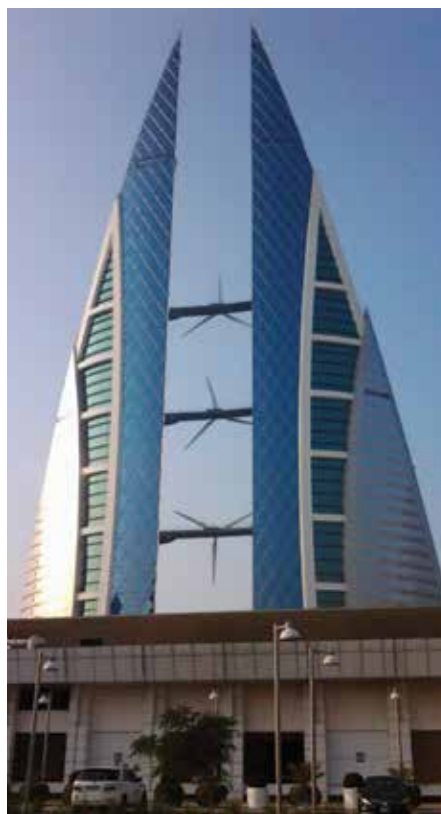
Figure 3. The wind turbines of the Bahrain World Trade Center. (Source: Ciacho5 (Own work) [CC BY-SA 3.0 ( http://creativecommons.org/licenses/by-sa/3.0/ )], via Wikimedia Commons)
