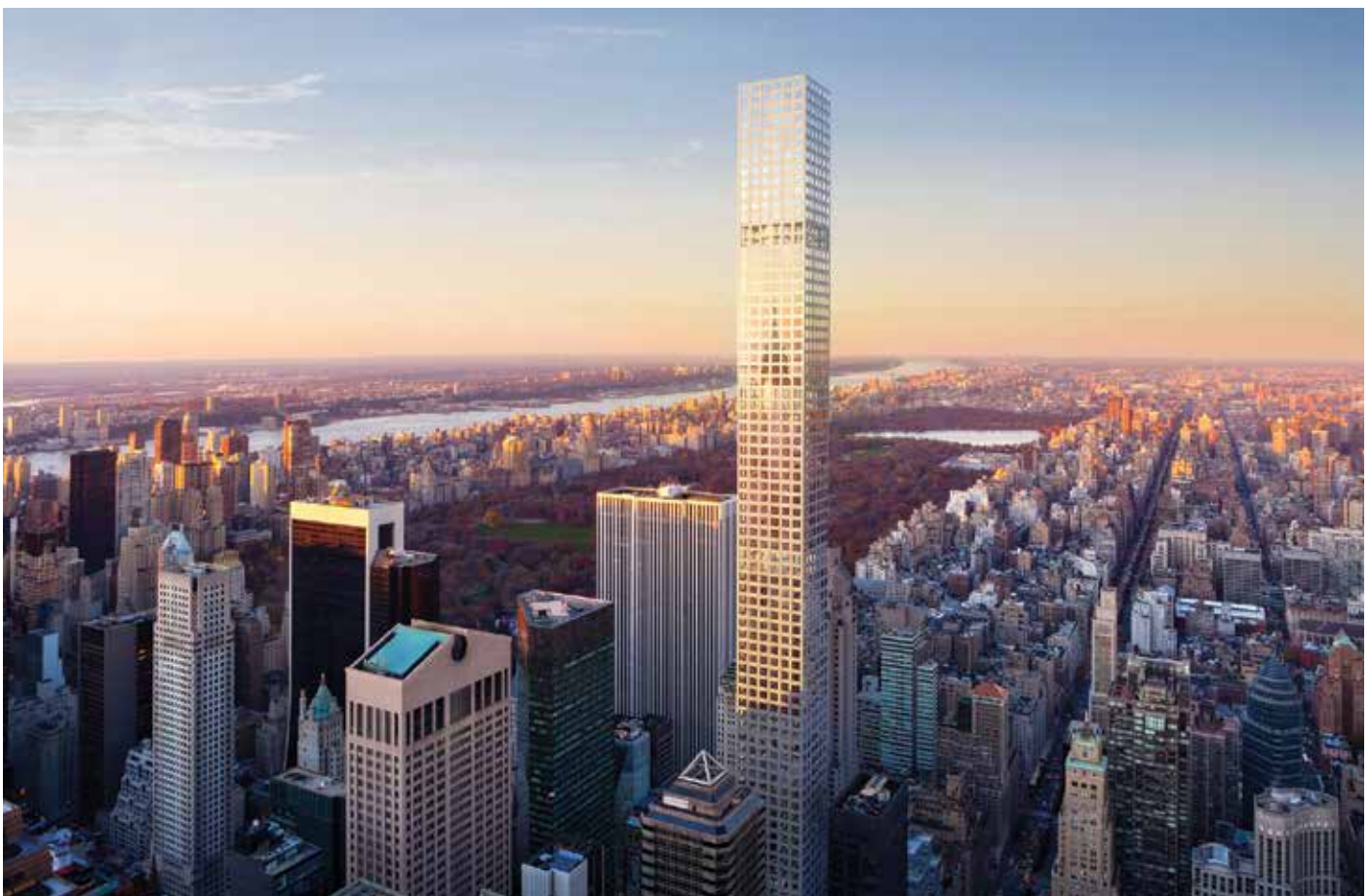
Figure 1. View from southeast
