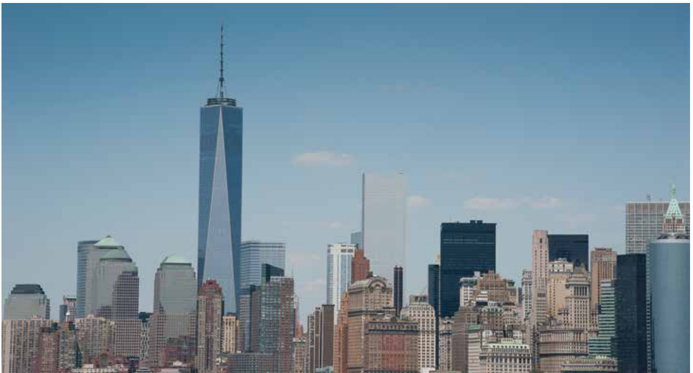
Figure 1. View of One World Trade Center from the East River (Source: WSP Group)
