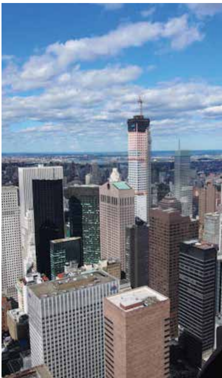
Figure 3. 432 Park Avenue during construction (Source: WSP Group)
