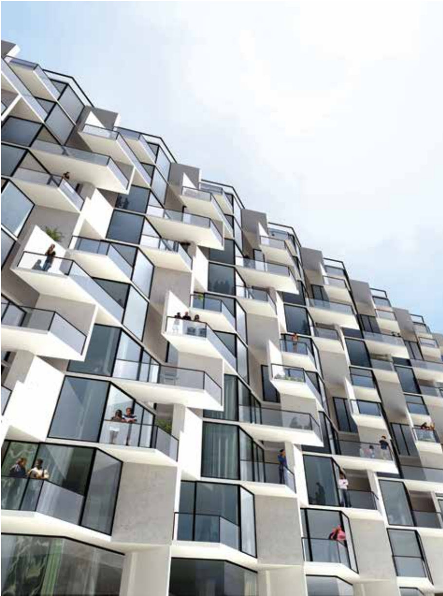
Figure 2. City Hyde Park's south-facing balconies offer opportunities for social interaction. (Source: Studio Gang Architects)
