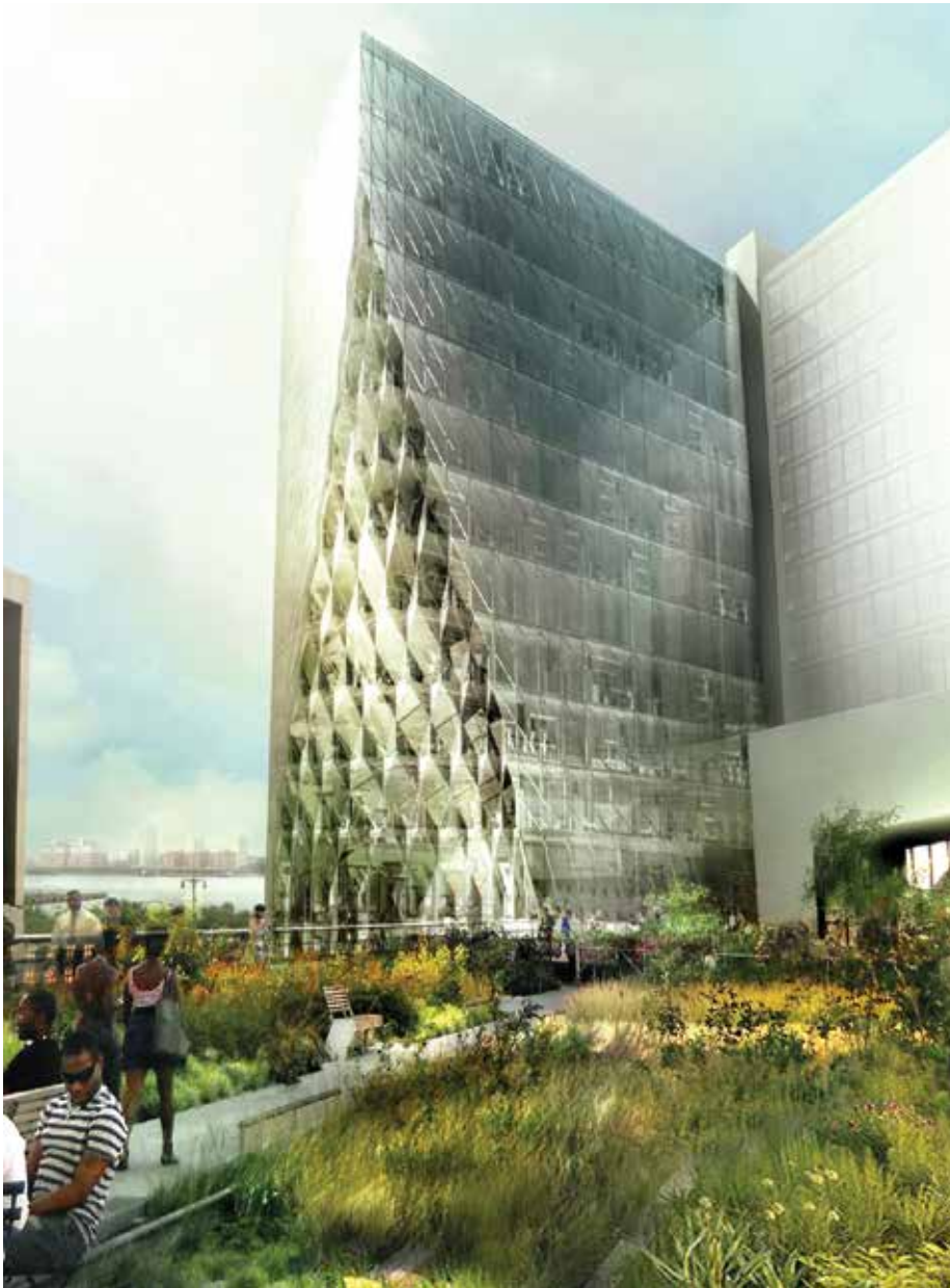
Figure 5. The shape of the Solar Carve Tower brings 200 more hours of daylight (annually) to the High Line Park than a building adhering to NYC zoning regulations. (Source: Studio Gang Architects)
