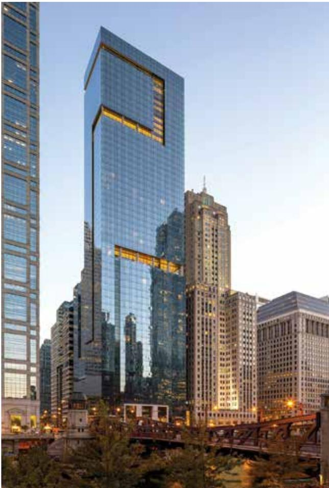
Figure 12. The executed building, with ribbon creating breaks at key program elements. Only the north east corner continues across both podium and tower (Source: Lester Ali)
