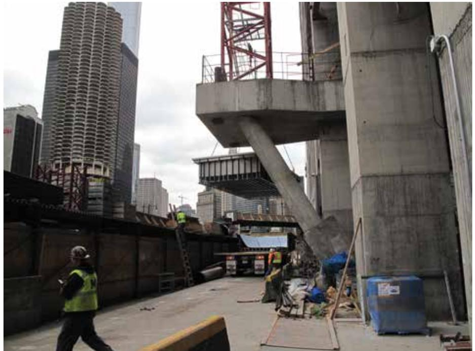
Figure 14. Crane "diving board", with swimming pool lift beyond (Source: Handel Architects)
