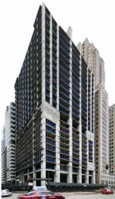
Figure 2. The existing structure, encompassing 25 floors of concrete slab above grade (Source: Handel Architects)
