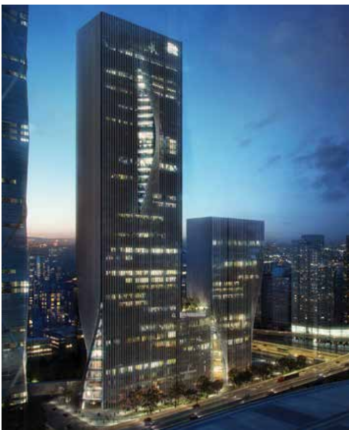
Figure 5. Shenzhen International Energy Mansion in Shenzhen, China (Source: BIG & Glessner)
