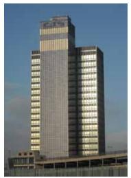
Figure 5. CIS Tower, Manchester – solar panel cladding. ⊕⊕@Gene Hunt
