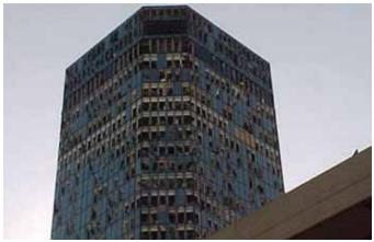
Figure 2. Bank One Tower, Forth Worth damaged by tornado in 2000. © Jesse Rangel
