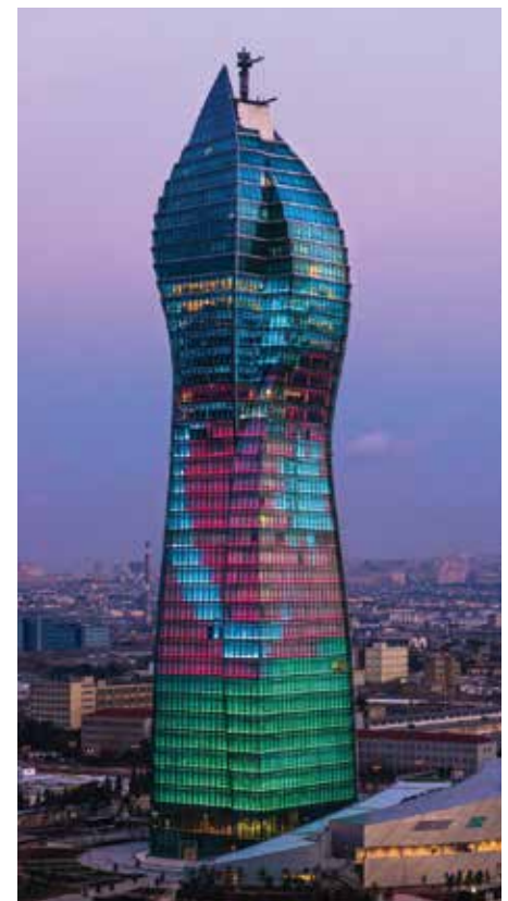
Figure 11. LED Lighting (Source: Heerim Architects & Planners)
