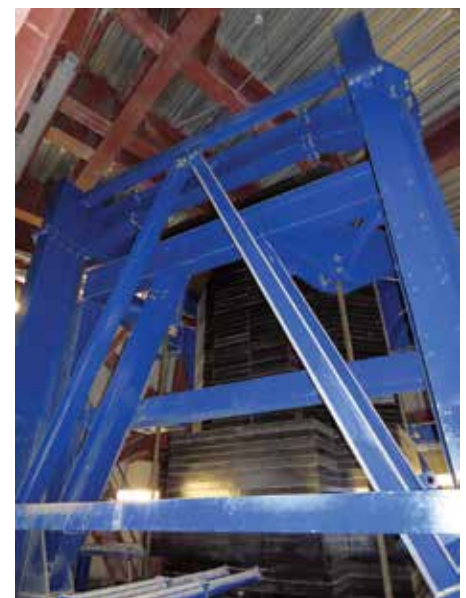
Figure 13. Tuned Mass Damper (Source: Heerim Architects & Planners)
