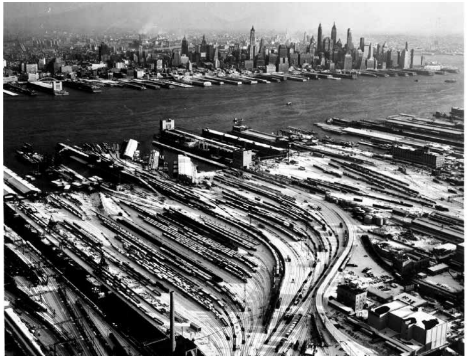
Figure 6. Freight rail era waterfront, now the Newport project (Source: Jersey City Public Library)
