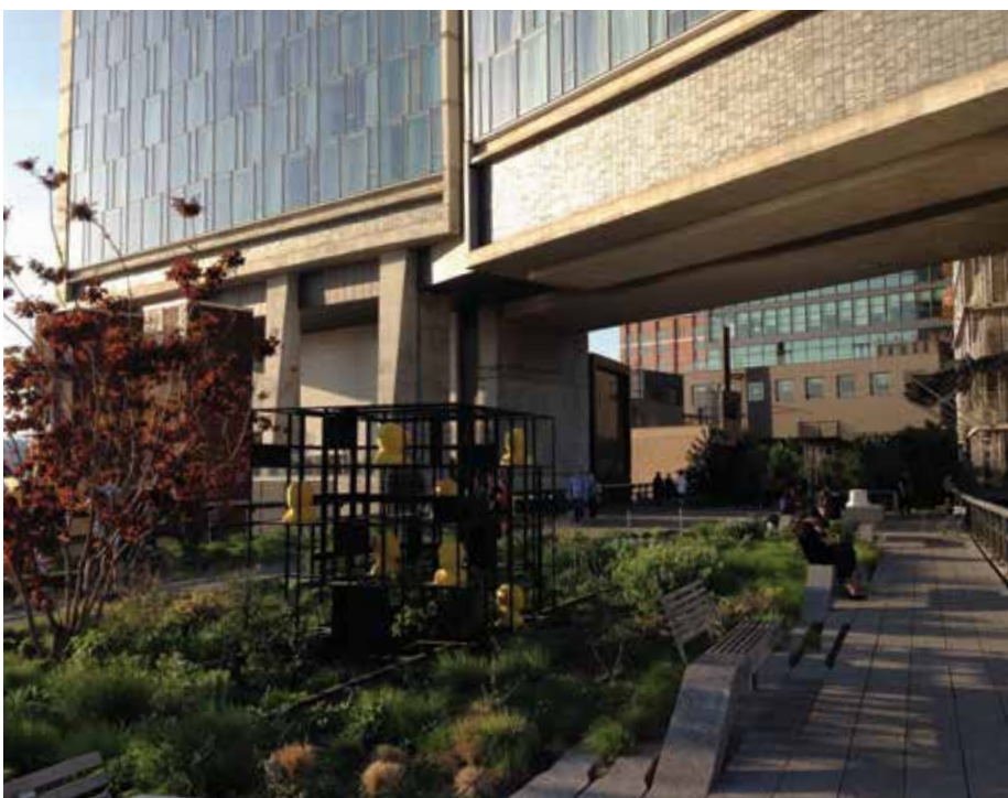
Figure 2. Hotel bridging over High Line (Source: Sabina Uffer)
