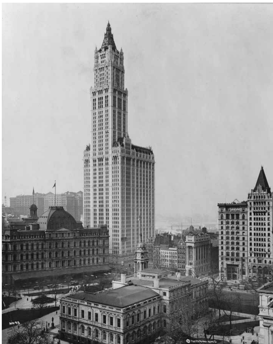
Figure 1. The Woolworth Building. (Source: Encyclopedia Structure, photographer Nicolas Janberg)
