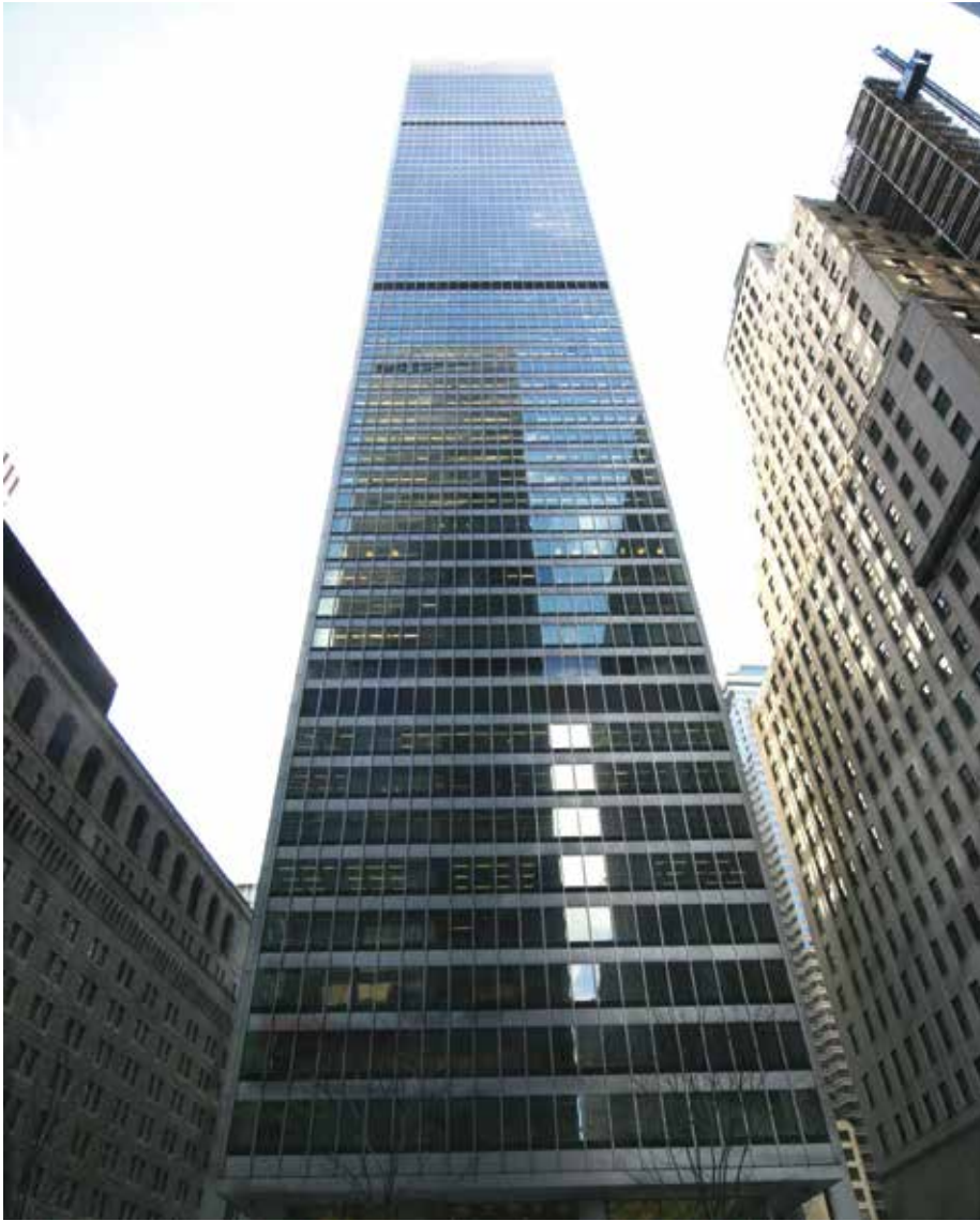
Figure 2. One Chase Manhattan Plaza, pictured, improves on previous 20th century floorplans by offering an off-center core and a glass façade, both of which improve daylight and visual connectivity (Source: New York City Landmarks Preservation Commission)
