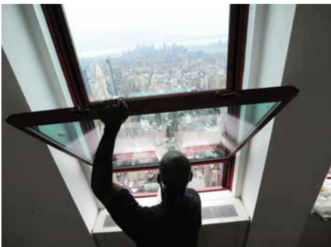
Figure 4. Window Replace 3 (Source: Empire State Realty Trust)
