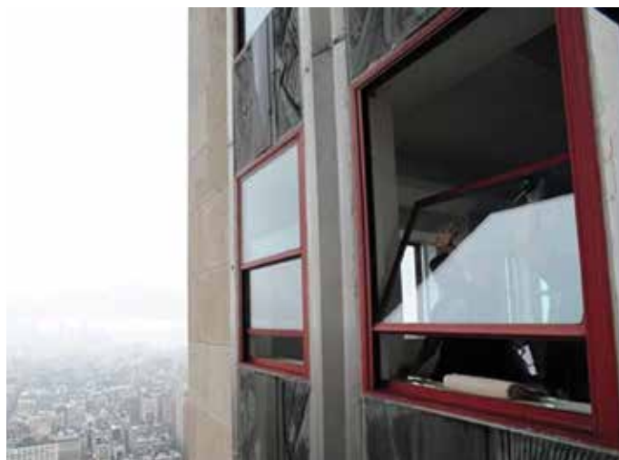
Figure 5. Window Replacement (Source: Empire State Realty Trust)
